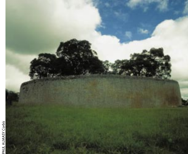
GREAT ENCLOSURE , shown here from the opposite side of the photograph on pages 94 and 95, perhaps served as the royal quarters of Great Zimbabwe. The structure was built during the city's heyday; its surrounding wall is 800 feet long and comprises an estimated one million stone blocks.
