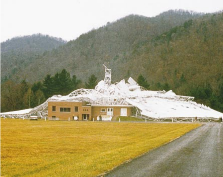
when a metal plate in the main support gave way. The $75-million replacement, now under construction, will be a paraboloid 110 by 100 meters; unlike traditional circular dishes, the new telescope will not have any support struts that block its view of the sky.
