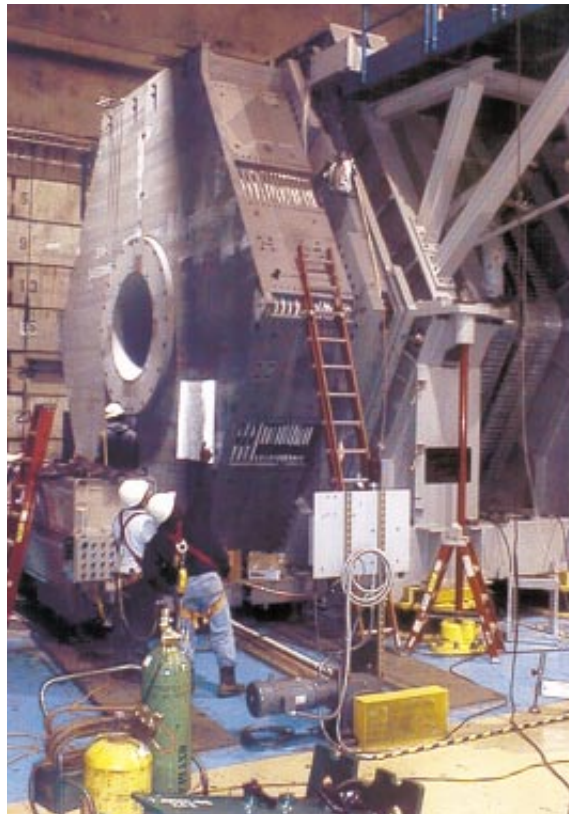
BABAR DETECTOR at Stanford University, being built by a collaboration from nine nations, will capture the decays of B mesons in charge-parity studies.
