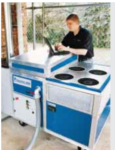
FUEL-CELL-POWERED HOME ( above ) in Latham, N.Y., gets its electricity from a refrigerator-size unit near the garage ( above right and at left ). The fuel cell, which is a variety known as proton-exchange membrane, supplies seven kilowatts—enough to meet much of the home's needs except during peak demand.
