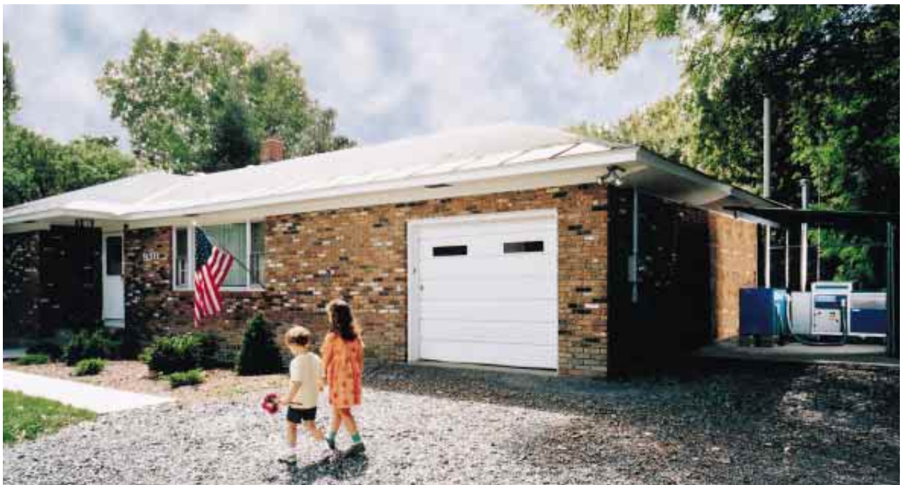
FUEL-CELL-POWERED HOME ( above ) in Latham, N.Y., gets its electricity from a refrigerator-size unit near the garage ( above right and at left ). The fuel cell, which is a variety known as proton-exchange membrane, supplies seven kilowatts—enough to meet much of the home's needs except during peak demand.
