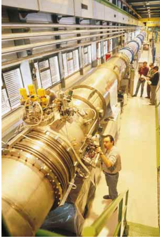
SUPERCONDUCTING MAGNET test string is laid out in the assembly hall; 1,232 such magnets will bend the trajectory of the two proton beams to follow the curve of the accelerator's tunnel.
