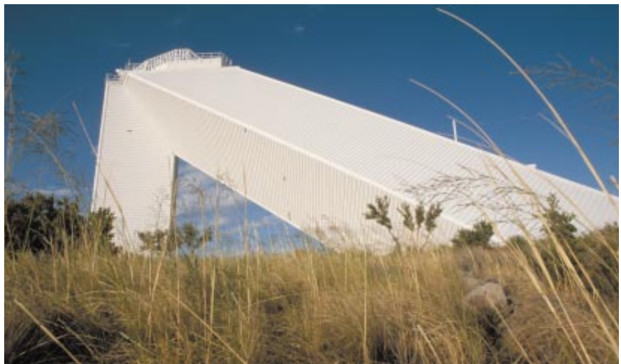
McMATH-PIERCE solar telescope's optical shaft runs underground, parallel to the axis of Earth.
