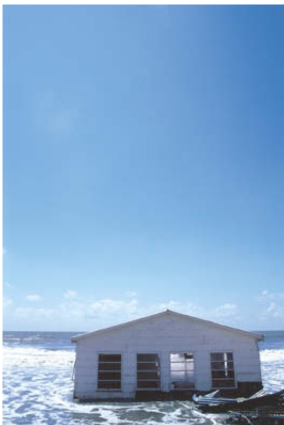
THIS OLD HOUSE floats on a barrier island that once protected the Mississippi Delta from the sea.
