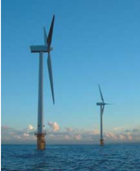
OFFSHORE WIND FARMS , such as these in the North Sea off the coast of Blyth in the U.K., are less likely to draw complaints of noise and unsightliness.
