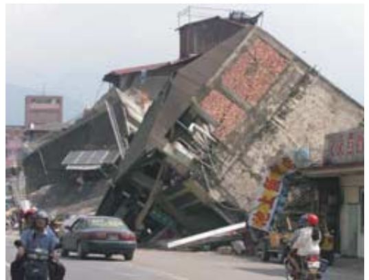
AFTERMATH: The devastation in Puli in central Taiwan, after a 7.3-magnitude earthquake and aftershocks on September 22, 1999.
