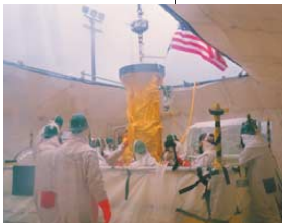
TOXIC BREW of radioactive waste lies just 10 feet below technicians working to replace a pump in a million-gallon storage tank at the Hanford site in Washington State.
