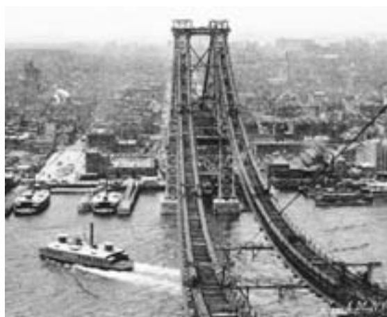
BUILDING the world’s longest suspension bridge, 1902
