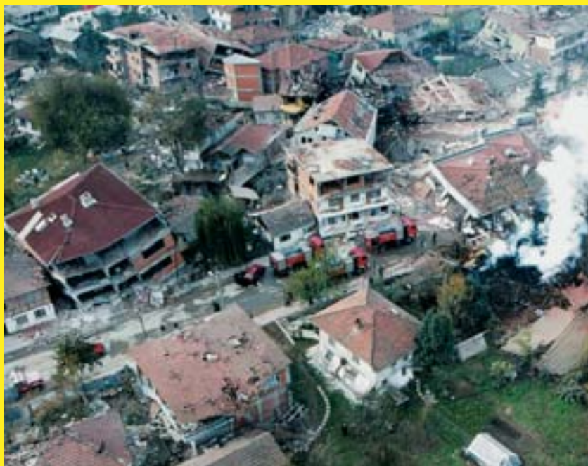
CRUMPLED BUILDINGS dot Düzce, Turkey, in the wake of a major tremor that struck in November 1999. Some scientists suspect that this disaster was triggered by an earlier shock near Izmit.
