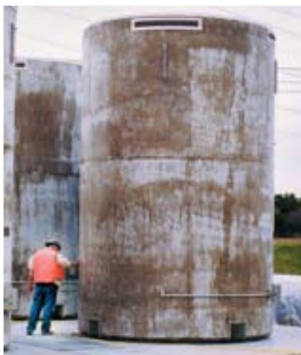
HIGH-LEVEL nuclear waste produced by power-generation plants finds a temporary home in on-site storage systems.
