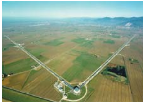
VIRGO INTERFEROMETER is built on a layer of sediment in the alluvial plain of the Arno River in Cascina near Pisa, Italy. VIRGO’s designers chose this site because of its low level of microseismicity.
