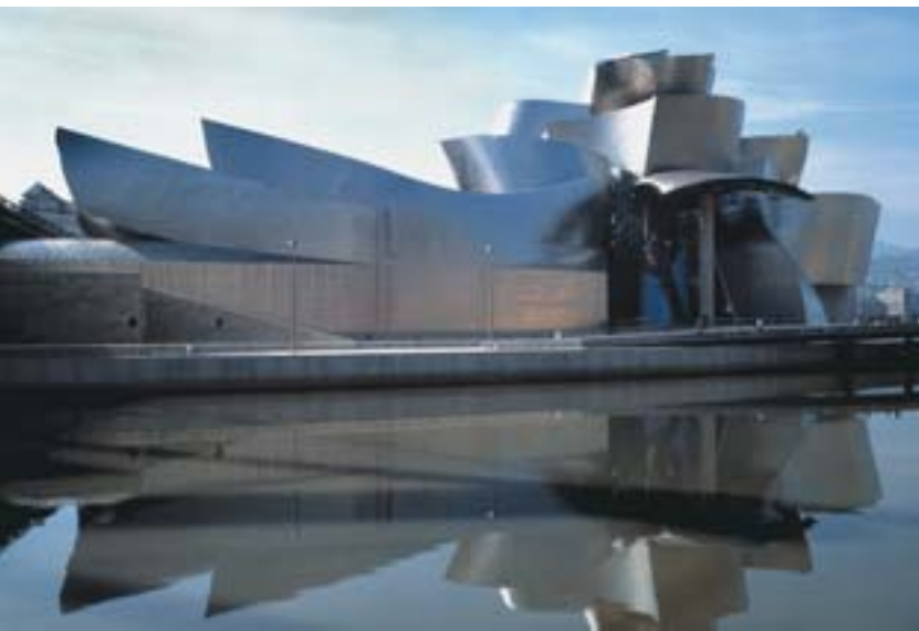
TITANIUM SHEATHES the Guggenheim Museum Bilbao in Spain. If the metal were cheaper, designers and engineers would use it more frequently.
