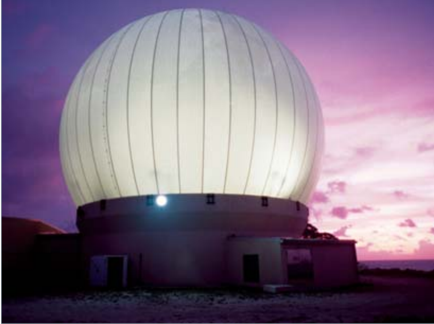
PROTOTYPE X-BAND RADAR located at Kwajalein Atoll was used in the tests of the missile defense system to track the mock warheads. Because the prototype's tracking abilities were limited, the interceptors also received location data from radar beacons placed on the warheads.
