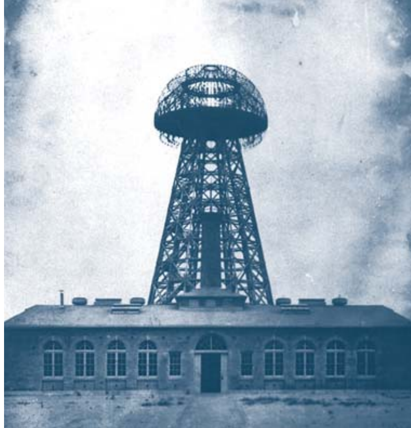
WARDENCLYFFE TOWER , at 187 feet tall, stood near the lab Tesla constructed in 1901 in what is now Shoreham, Long Island. The facility was intended both for transatlantic wireless communications and radio broadcasting, as well as for global transmission of electric power.
