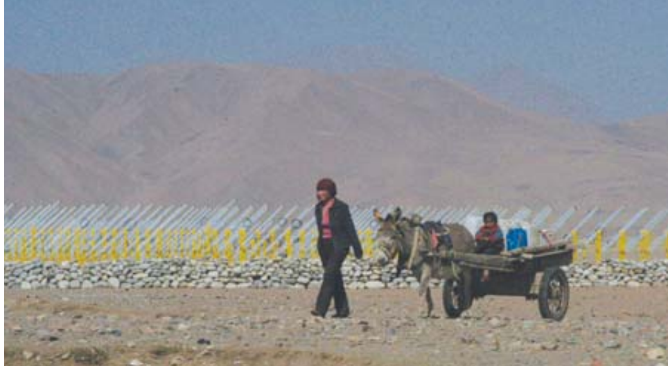
LOW-TECH RADIO TELESCOPE under construction in western China will use thousands of consumer television antennas and hundreds of cheap personal computers to slice through the fog that shrouded the infant universe.
