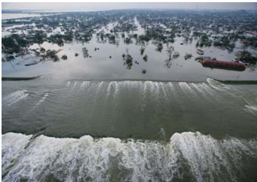
DROWNING CITY: Battered by the August 29 arrival of Hurricane Katrina, levees protecting New Orleans crumbled, such as this one along the Inner Harbor Navigational Canal. Tattered wetlands around the city offered little protection against stormy seas.
