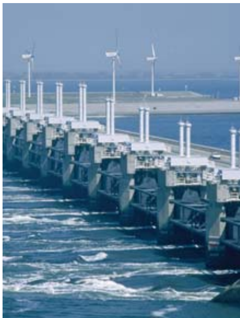
DUTCH LESSON: The Oosterschelde, a storm surge barrier in the Netherlands, allows the North Sea to mix with freshwater, thus helping to keep wetlands intact.
