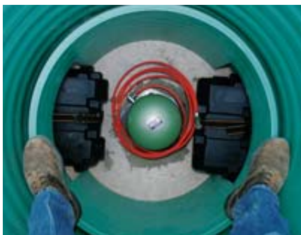
SEISMOMETER (green sphere) with supporting electronics (black) is sealed in a tank on a concrete pad to keep the device level. It is one of hundreds used by EarthScope.
