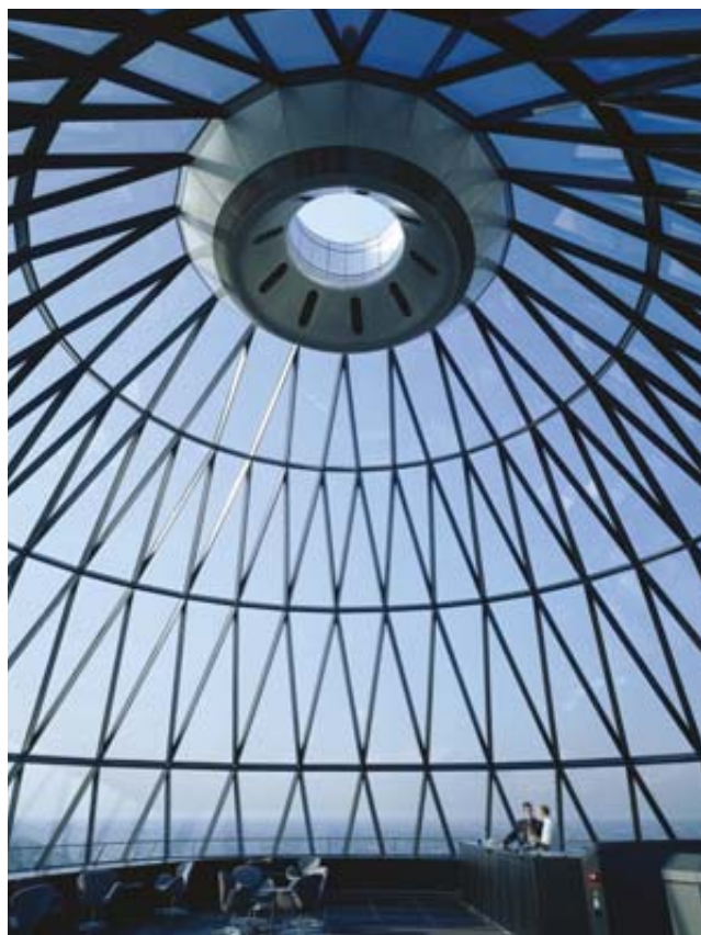
A huge glass spire formed in the shape of a chrysalis tops the Swiss Re building in London, finished in 2004. Wind flowing across its walls drives the ventilation system and diminishes air-conditioning needs.
