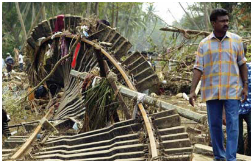
TWISTED RAILWAY TRACKS near Sri Lanka's southwestern coast community of Sinigame mark where the December 2004 tsunami derailed an eight-car passenger train, killing an estimated 1,500 people.
