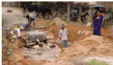
BIOGAS REACTOR , which consists of a well for fermenting dung, is being built in Tamil Nadu, India, as part of the World Cup's Green Goal program.
