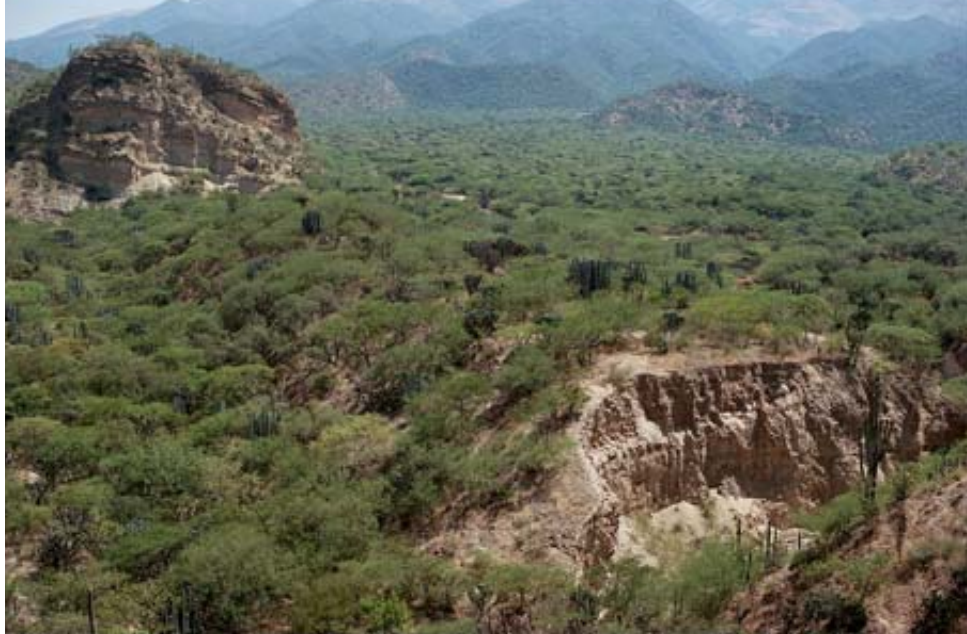
PURRÓN DAM (at lower right in photograph above) near Puebla, Mexico, is believed to be the largest water retention structure built in the Americas before the arrival of the Europeans. Construction began in 750 B.C. and continued at intervals until about A.D. 1150, when the dam stood almost 25 meters high and stretched 400 meters in length. The eroded southern profile of the dam (far right) dwarfs a six-foot-tall man.
