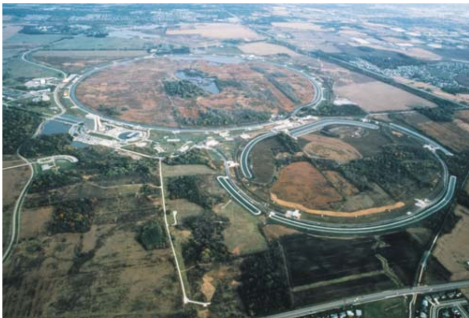
ON TOP: Fermilab's main injector ring ( foreground ) feeds accelerated particles to the Tevatron ring ( background ), which is two kilometers wide and sits 10 meters below ground. Particle collisions have yielded top quarks without their antimatter twins.
