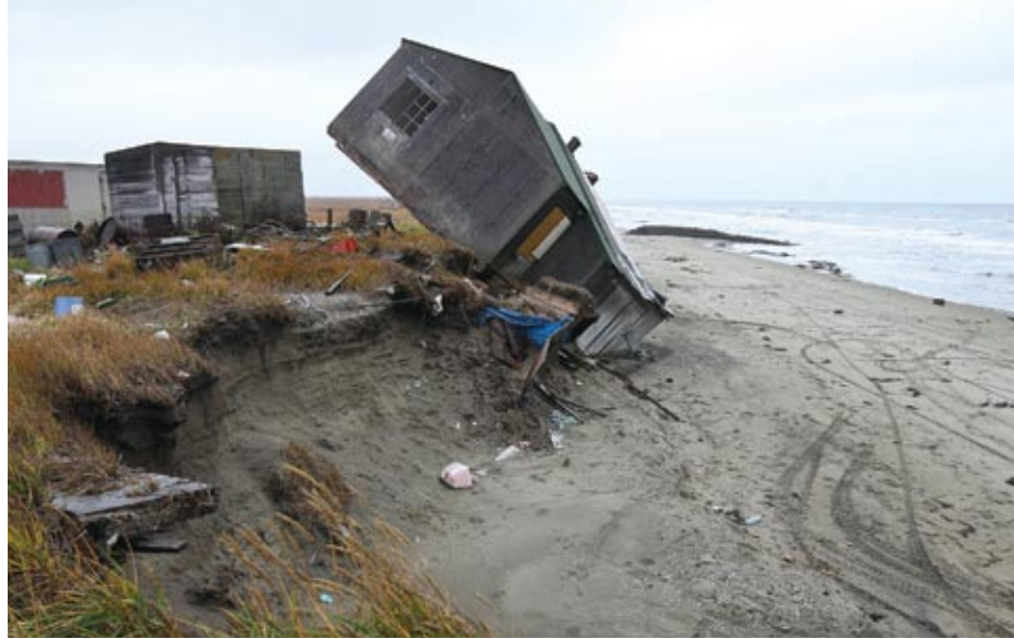
DEVASTATING COASTAL EROSION in the Alaskan village of Shishmaref, caused by the loss of permafrost and storm-buffering sea ice in a rapidly warming climate, is forcing the villagers to abandon their island homes and relocate to the mainland.
