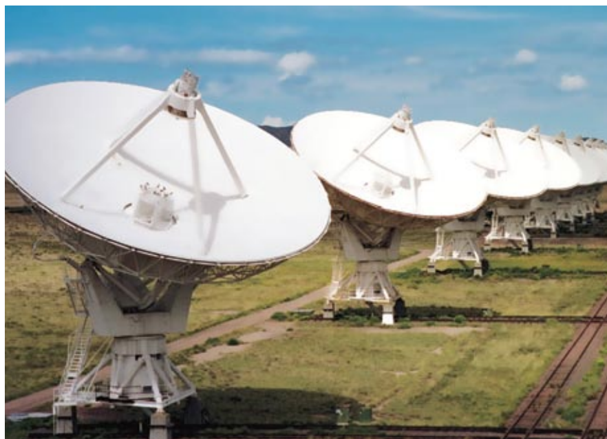
GETTING ENHANCED: The Very Large Array near Socorro, N.M., maintains 28 movable dishes that are each 25 meters in diameter. Various upgrades, to be completed by 2012, will dramatically boost the array's resolution, sensitivity and data-handling ability.
