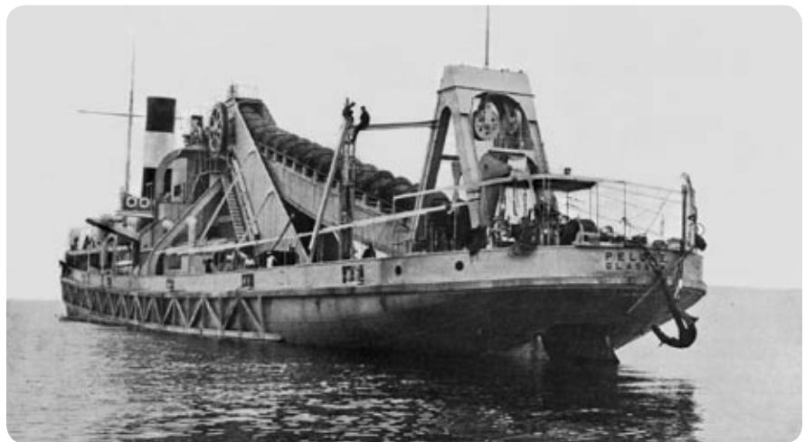
MACHINERY VS. MUD —the largest bucket dredger for the Suez Canal, 1908
