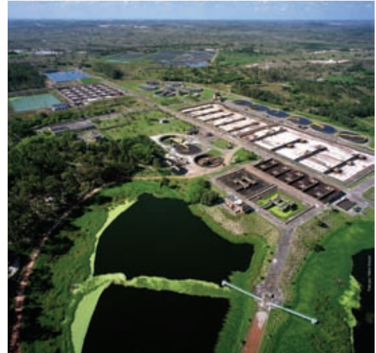
The Waste Water Treatment Plant of Cetrel
