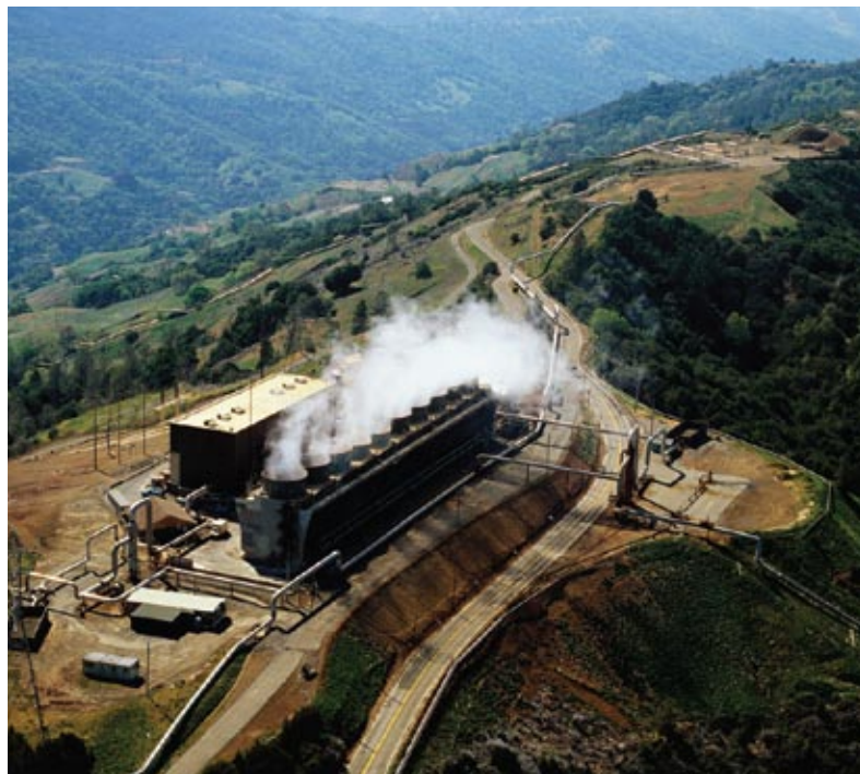
POWER PLANT near Santa Rosa, Calif., is fueled by underground steam. The emission is water vapor.
