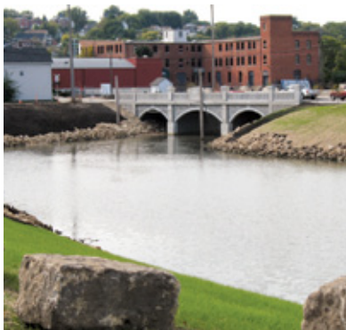
Banking on it: Dubuque, Iowa, opened a buried creek so that it will absorb water during storms instead of flooding town.
