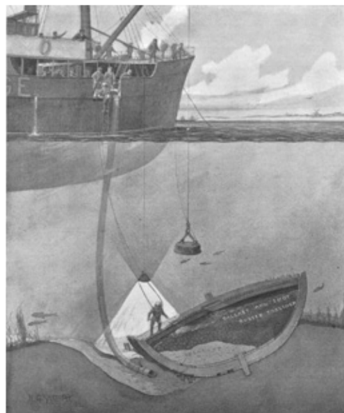
HEAVE-HO: Salvagers planned to use a powerful electromagnet to get at buried treasure, 1913
