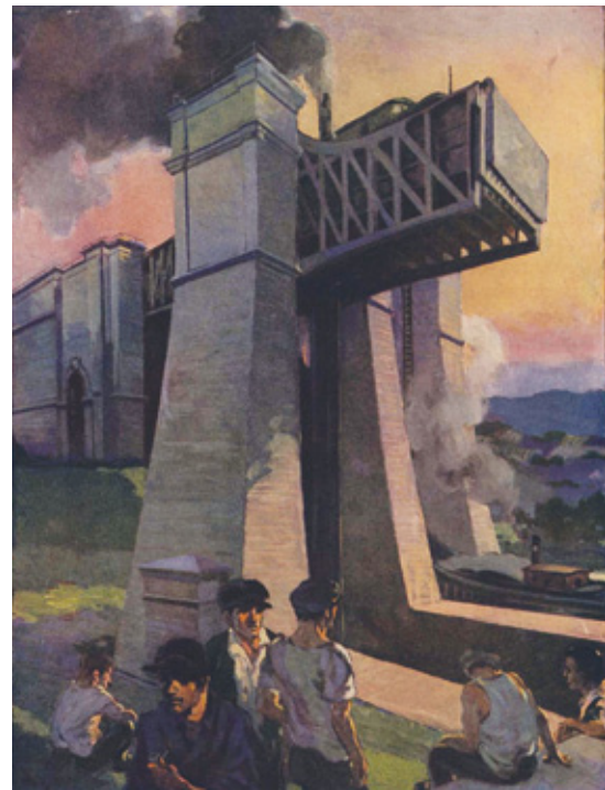
HYDRAULIC LIFT LOCK: This image graced the cover of the September 6, 1913, issue, which featured articles on several canals. The lock shown here, at Peterborough on the Trent-Severn Waterway in Canada, carries barges 65 feet straight up and down. It is still in use today.
