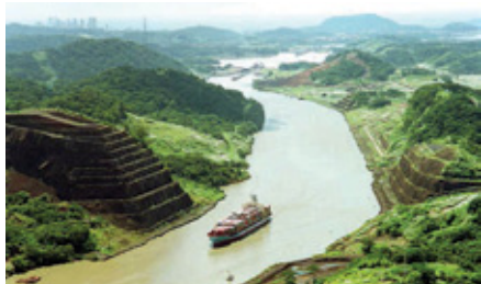
Gaillard Cut, Panama Canal
