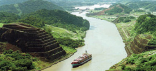
Caravan makes it your year to visit Panama and the Panama Canal! Photo: Gaillard Cut, Panama Canal
