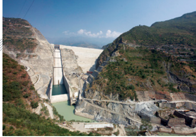
India’s Tehri Dam blocks Bhagirathi River, a main tributary of the Ganges.
