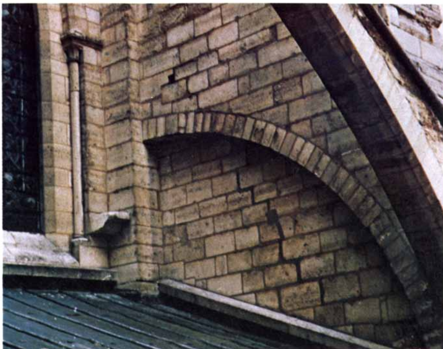
TWELFTH-CENTURY WALL BUTTRESS above the gallery on the south transept at the cathedral has embedded in its inner face an arch that probably repeats the arc of the original upper fliers, which supported the adjacent nave clerestory. This archaeological evidence suggests that the first flying buttresses abutted the clerestory at a point about halfway up the original windows, well below the roof. In the 13th century the upper fliers were replaced by huge flying buttresses spanning both side aisles, and the clerestory windows were enlarged.
