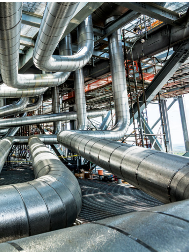
KEMPER HAS REQUIRED 172 miles of tangled pipes, 40,000 tons of steel and two giant gasifiers (one at center, above right) to convert dirty coal into a cleaner-burning gas and to prevent the CO 2 by-product from being dumped into the atmosphere.
