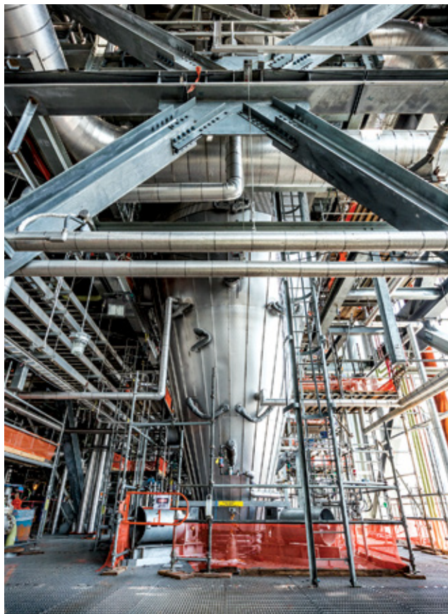
KEMPER HAS REQUIRED 172 miles of tangled pipes, 40,000 tons of steel and two giant gasifiers (one at center, above right) to convert dirty coal into a cleaner-burning gas and to prevent the CO 2 by-product from being dumped into the atmosphere.
