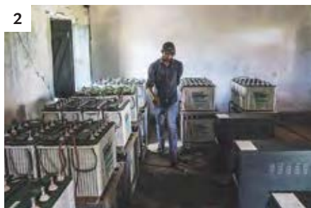
MICROGRIDS can power villages that electric transmission lines do not reach. Solar panels feed a local microgrid in one village (1). Batteries store solar power for another microgrid (2).
