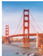
Day 1, 2 Golden Gate Bridge
