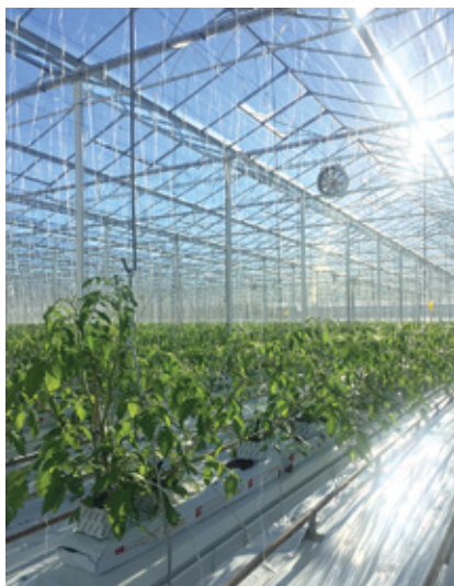
VANCOUVER burns methane collected at landfills to produce heat that warms tomato greenhouses run by Village Farms.
