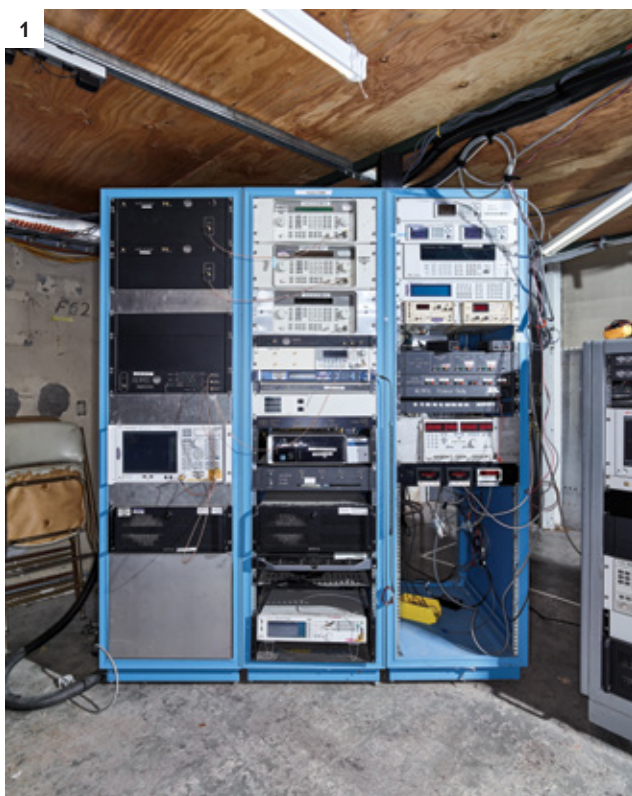
1 EQUIPMENT RACKS house ADMX's room-temperature microwave electronics (1). Engineers study sensor data from the experiment (2).
