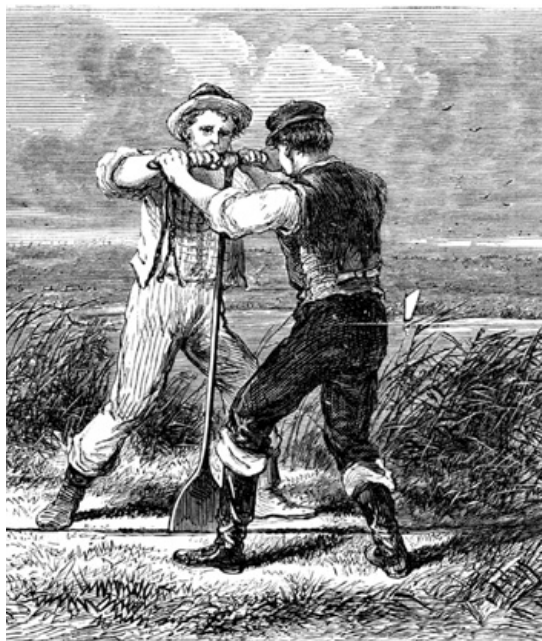
1868: Two workmen “chisel” a trench for an iron plate to help drain swamps in New Jersey.
