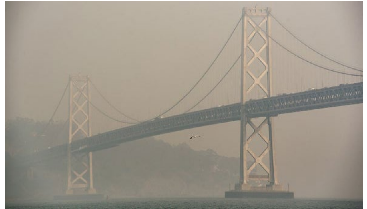
Bay Bridge is obscured as smoke from the Camp Fire fills the air in San Francisco on November 15, 2018.
