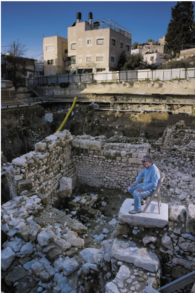
EXCAVATION in a former parking lot just south of the Old City reveals evidence from the sixth century B.C.E. to the early Muslim period a millennium later (left), including a gold earring from the Hellenistic era in the third century B.C.E. (right).
