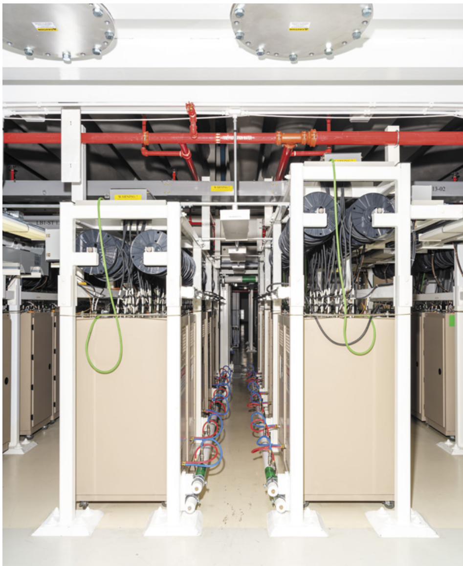
INSIDE THE LASER BAY , high-voltage instruments control the propagation of the laser beams through the amplifiers.
