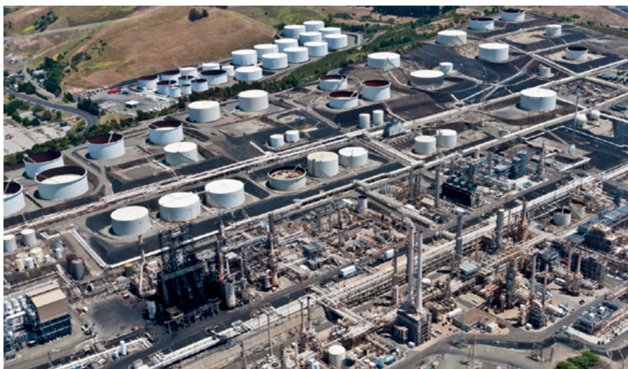
The petroleum company Phillips 66's oil refinery in Rodeo, California.
