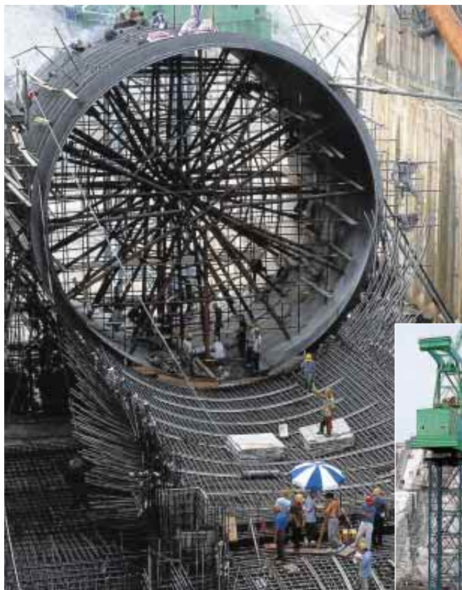
FEEDING THE TURBINES: Huge water intakes ( left ) will divert water from the Yangtze River to one of 26 gigantic turbines. At full capacity the dam will generate 18,200 megawatts, making it the biggest hydropower producer in the world. The intakes are placed about halfway up the dam's eventual 60-story height ( below ).
