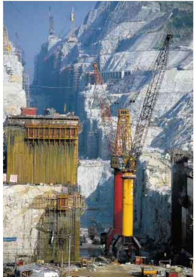
GIGANTIC LOCK: Matching the dam in scale, an enormous five-step lock ( right ) is being carved from granite on the river's left bank. The chambers of the lock will be lined with concrete, and when completed it will lift 3,300-ton ships 285 feet, making it the largest such system in the world.
