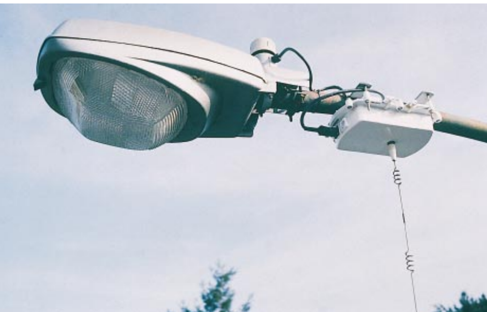
RADIO TRANSMITTERS inconspicuously placed on light poles a quarter mile apart have already established a wireless communications network over sections of Seattle, San Francisco and Washington, D.C. A wireless modem in communication with these devices, which in turn interface with wired access points, enables users of the network (built by Metricom) to access information far from telephone lines.
