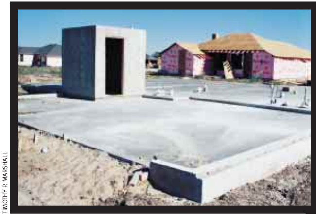
STORM BUNKER: Steel-reinforced concrete “safe rooms” can sometimes provide protection against the fury of tornado-strength winds.
