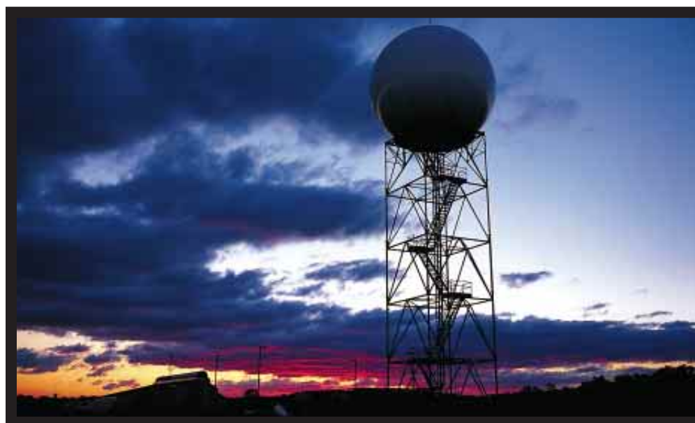
TOP-OF-THE-LINE EQUIPMENT: The Doppler radar tower (above) near Washington Dulles Airport is one of the workhorses intended to increase the accuracy and timeliness of weather forecasts. The opposite page shows the early morning launch of a weather balloon.
